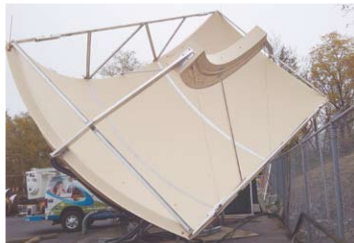
Antietam technicians (above) working on the new master satellite dish are dwarfed by the size of the 6,000 pound piece of equipment that was put in place with a giant crane. Below is the finished product.
