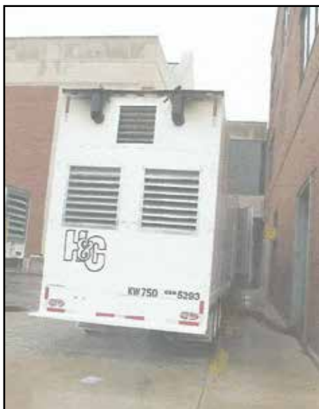
Truck-sized generators provide the Tribune with electricity during a three day power outage.
